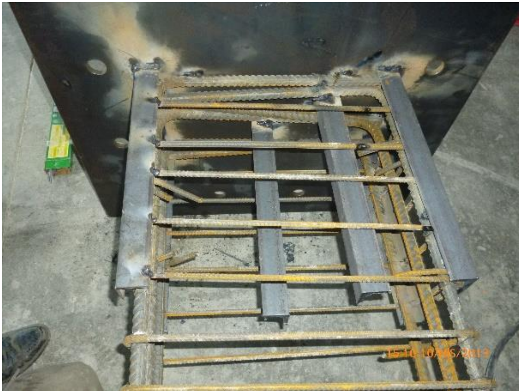
Figure 4.18. Detail of column bottom plate
