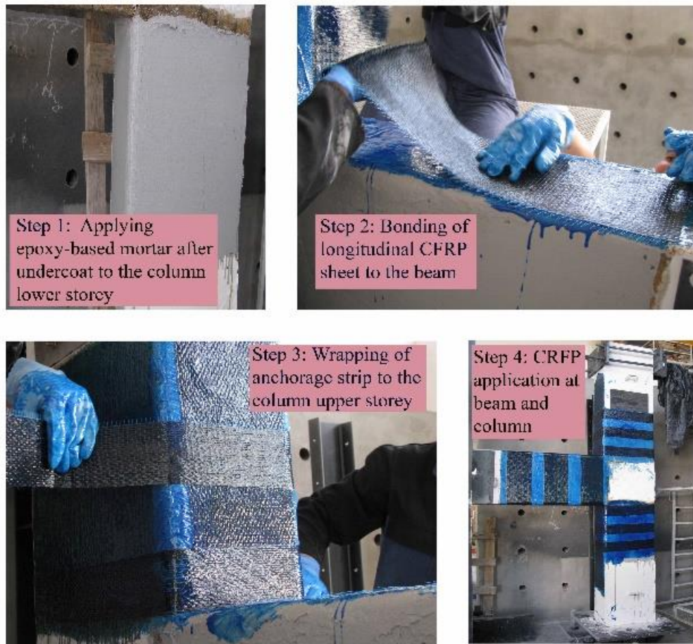
Figure 4.13. The repair process of EJ-1-R as shown in Figure 4.12
