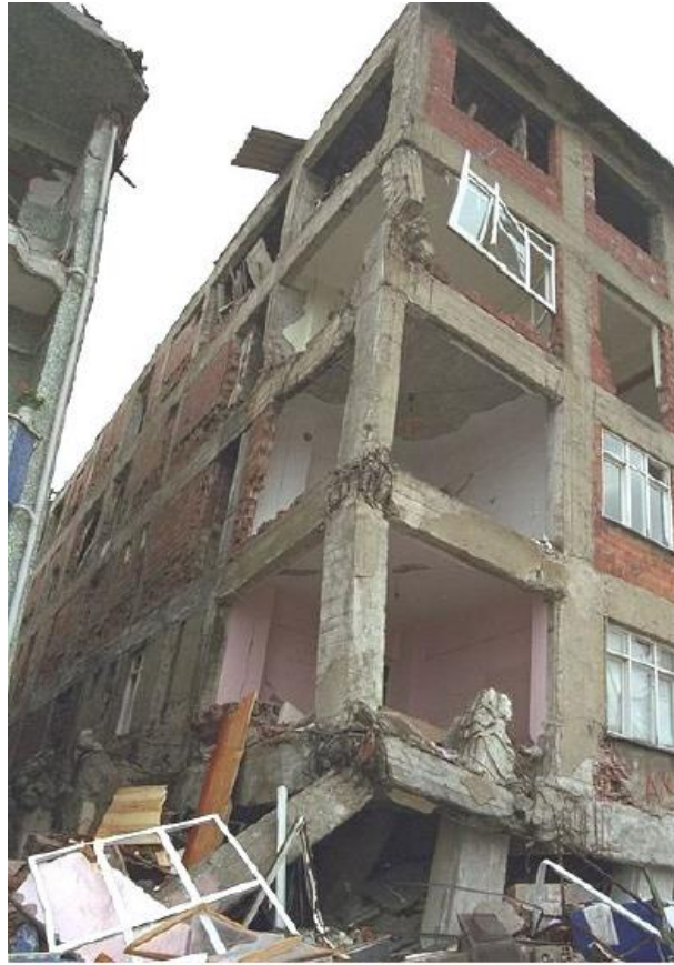
Figure 2.8. Adapazarı-Turkey Earthquake (1999), Photo credit: NISEE [15]
