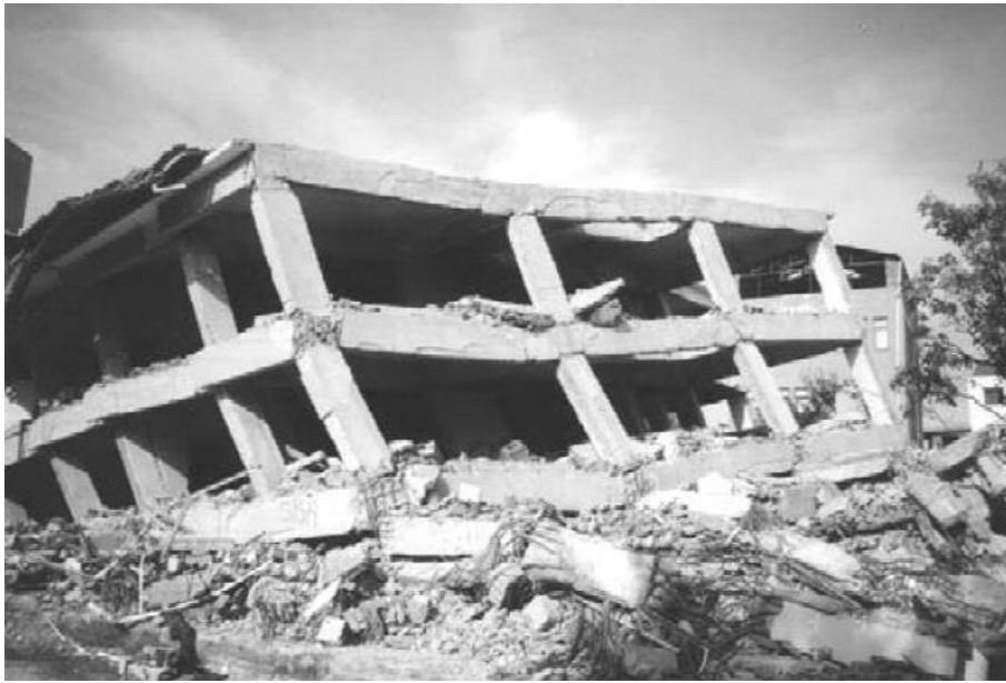
Figure 2.5. Collapsed building in Adapazarı-Turkey Earthquake (1999) [13]
