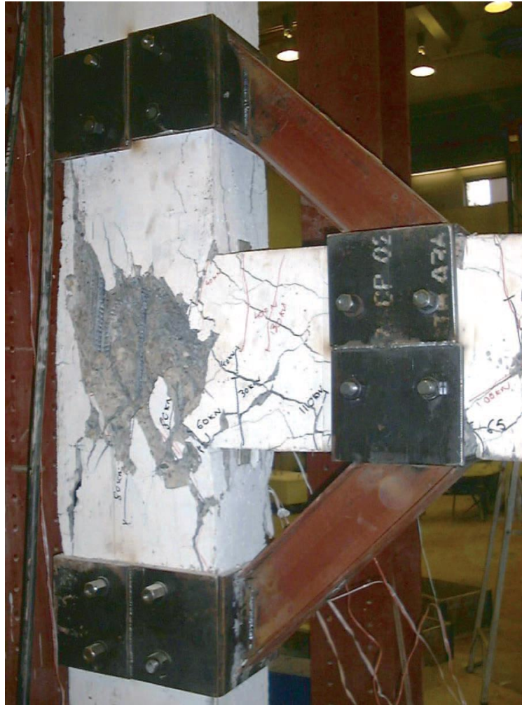
Figure 3.15. Crack patterns in retrofitted specimen [29]
