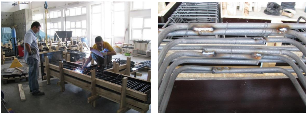
Figure 4.8. Welding of beam hooks
