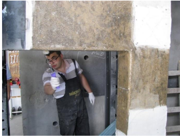
Figure 4.9. Application of MBT-MBrace® Primer
