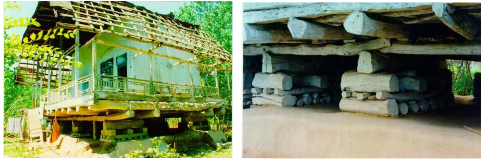
Figure 1.7. Decoupling the structure from the ground, Iran [5]
