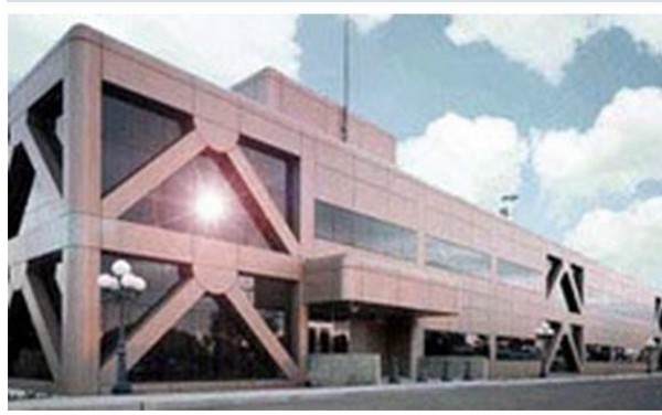
Figure 1.11. Caltrans Traffic Management Center, Kearney Mesa, California [10]
