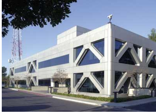
Figure 1.9. Los Angeles County Fire Command & Control Facility, California [8]
