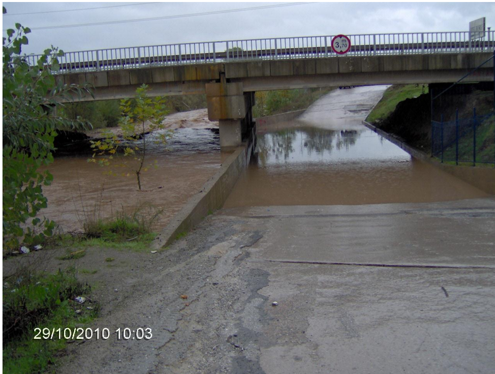
Figure 3.17 Downstream channel section at 11+400 km
