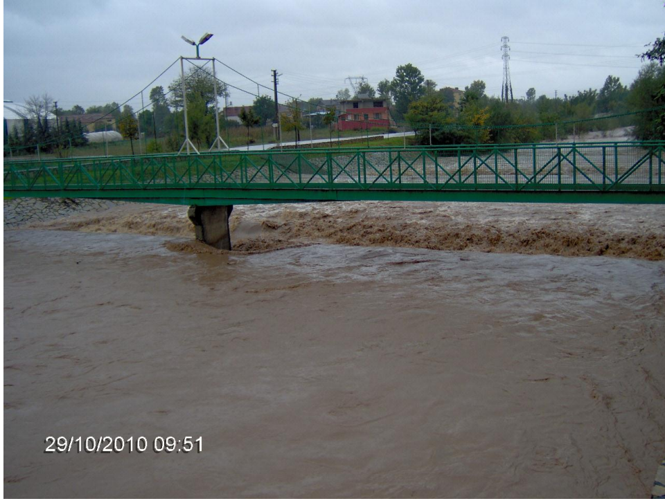
Figure 3.16 Downstream channel section at 7+800 km
