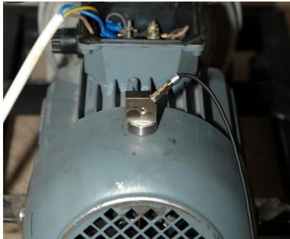
Figure 3.5. Accelerometer and its position on fan cover of the motor
