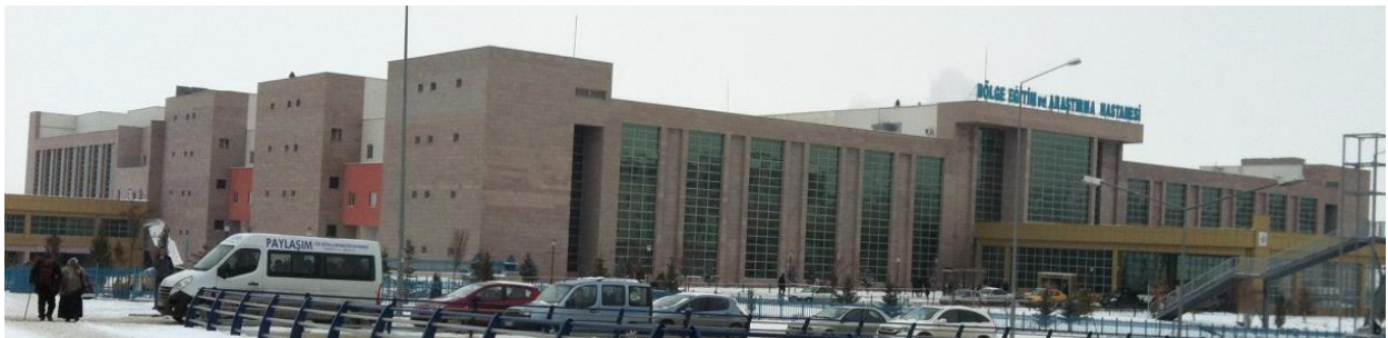
Figure 2. General view of the Erzurum Hospital
