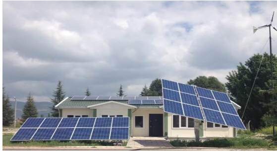
Fig 1. The Installed fixed (left side) and sun tracking solar PV panels (right side) with same capacity (3 kW) in Iki Eylul Campus of Anadolu University, Eskisehir, Turkey.
