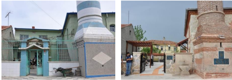
Figure 3-4. Hacı Hasan Mosque, before and after the restoration.
