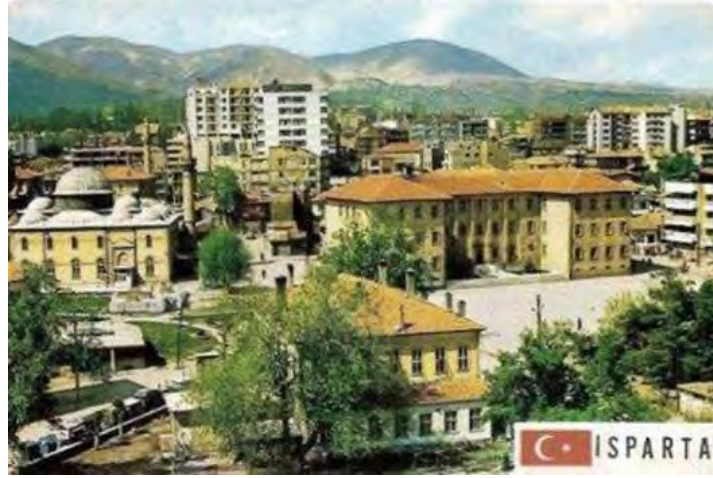
Figure 11. View of Governor's Building and its surroundings in the 1980s (Source: Website of Haber 32, 2014).
