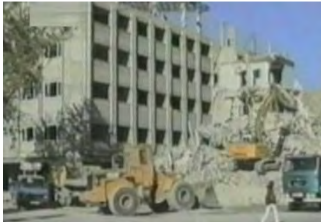
Figure 20. Pulling Down of Ranging Stores in 1992 (Source: Website of News 32, 2014).
