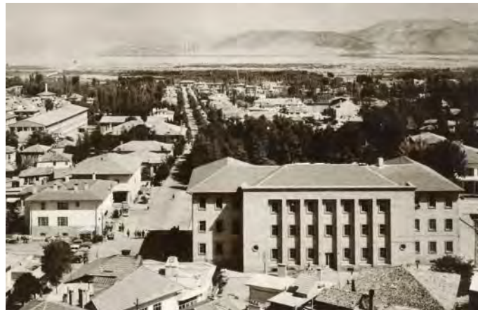
Figure 15. Back elevation of Governor's Building in 1970 (Source: Foto Venüs, 2011).
