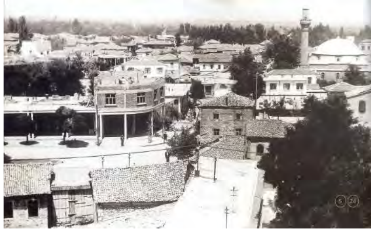
Figure 8. Ranging Stores and Mimar Sinan Mosque in 1955 (Source: Anonymous, 2001).
