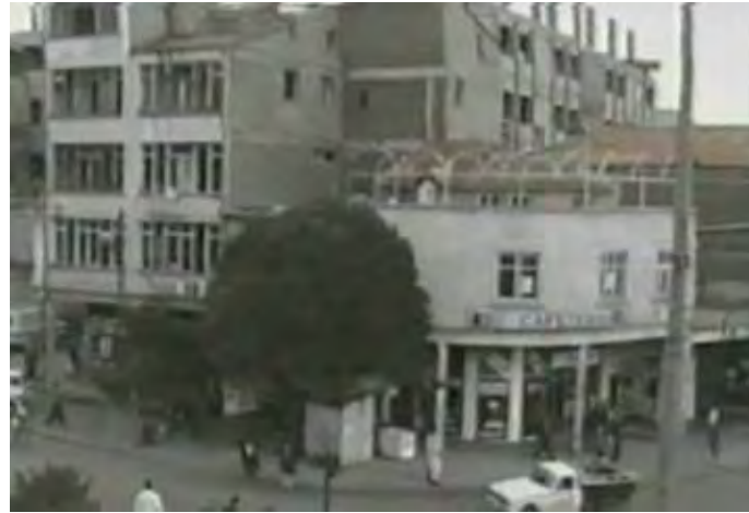
Figure 18. View of Ranging Stores Before Pulled Down in 1990 (Source: Website of Haber 32, 2014).
