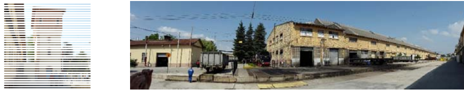
Figure 7. Tulomsas factory water tower (left), production buildings (right). Source: top right Kandemir's private collection, 2015
