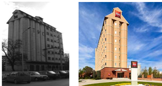
Figure 10: Grain silo before (2009) and after (today) adaptation process [22, 23]
